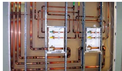
Typical commercial medical gas installation rough-in.
